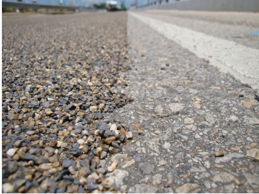
Figure 3. Photograph. HFST post installation.
