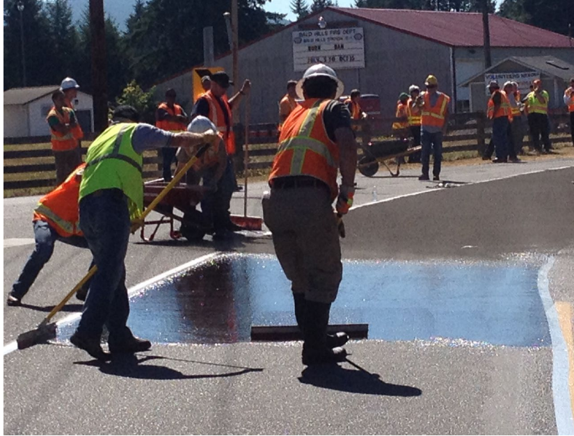
Figure 1. Photograph. Manual HFST installation.
