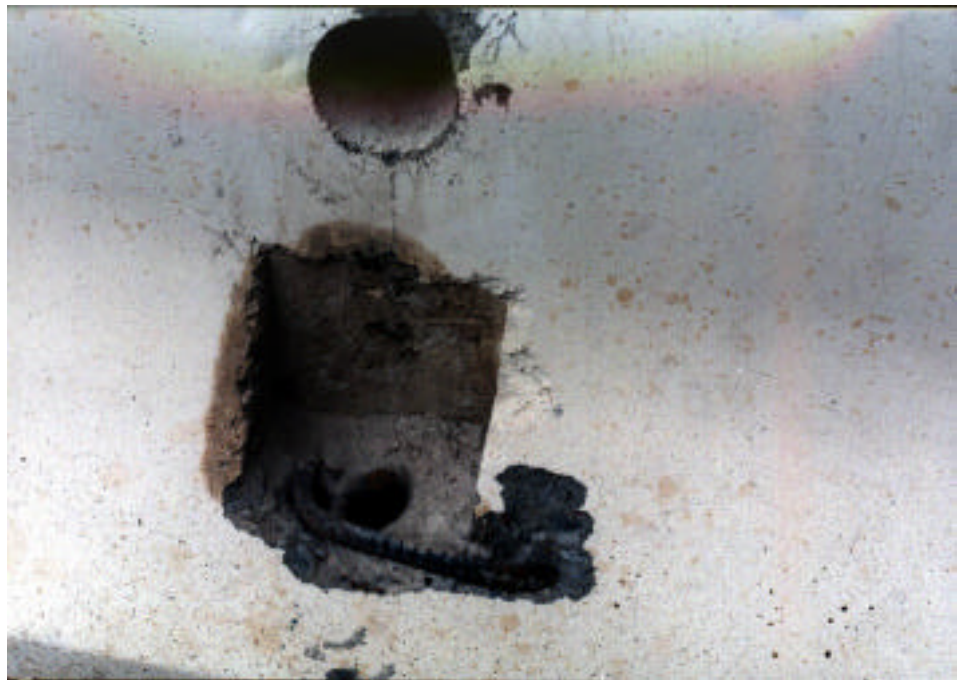
Figure 2-3 - Exposed Rebar
