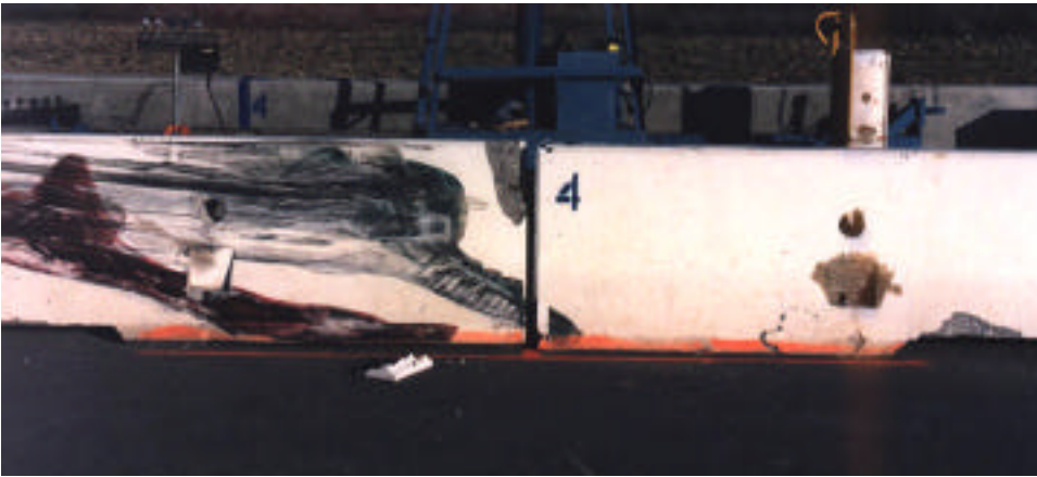
Figure 2-11 - Post Impact View of Barrier
