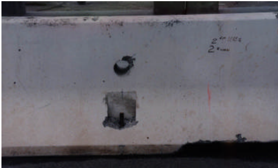
Figure 2-2 - View of Anchor Stake in Barrier
