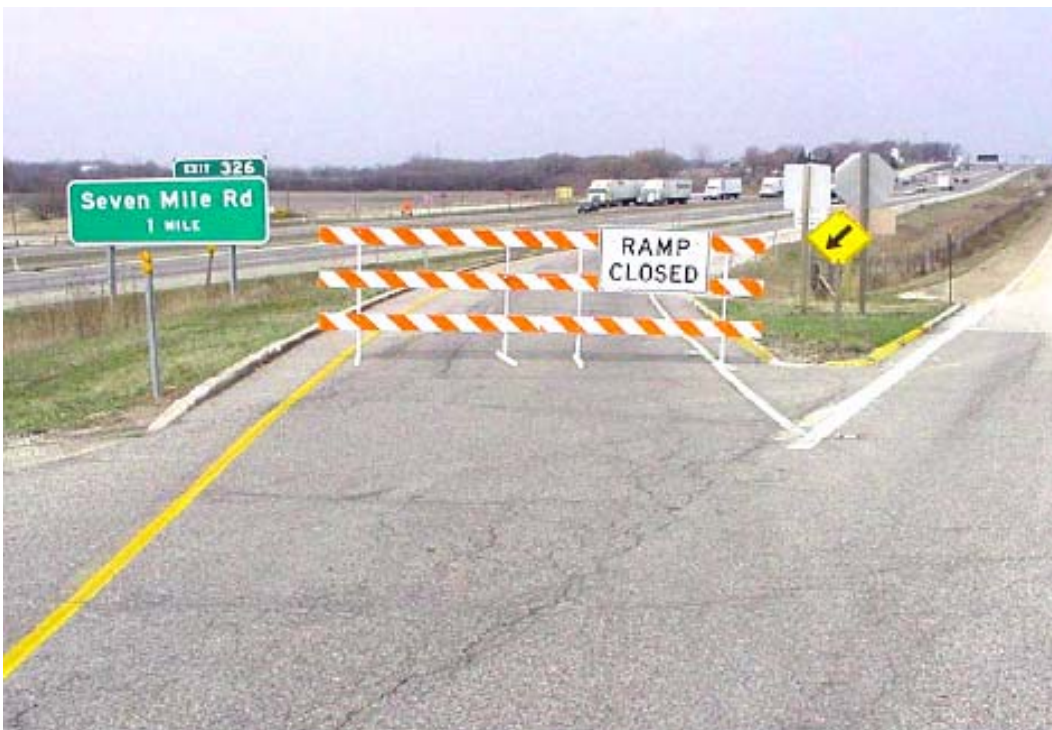
Figure 10-21: Type III Barricade (Deployed) 28
