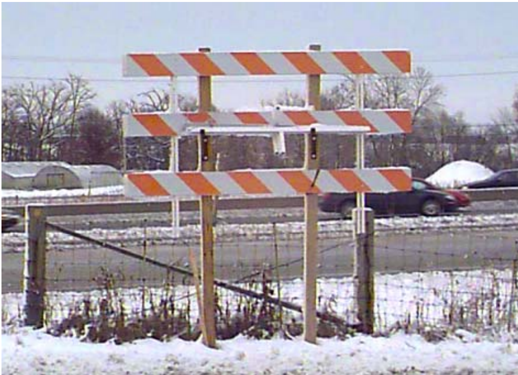
Figure 10-20: Type III Barricade (Stored Position) 28
