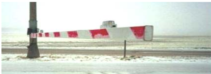
Figure 10-23: Vertical Swing Arm Traffic Gate (Closed Position) 29
